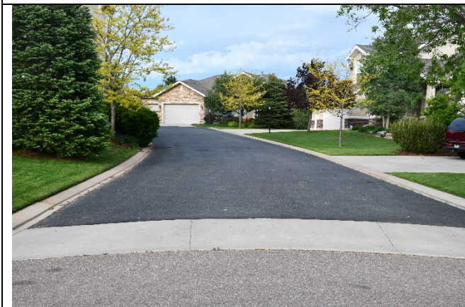
Photo #30 – Pavement – Sage Hill
